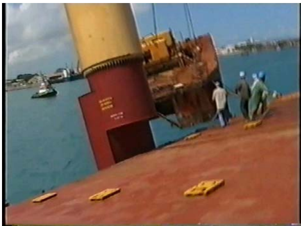
Moments before cranes ordered to slack the barge into the water
