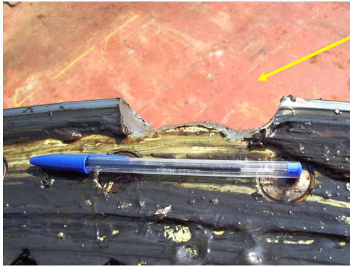
Damage to slew gear showing area through which bearings had torn
