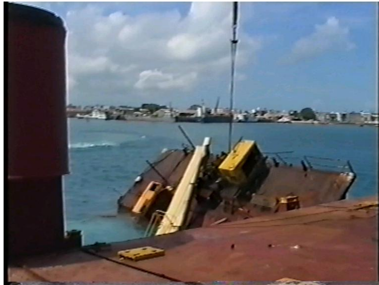
Final resting place of Number 2 crane in the sea, supported on the barge
