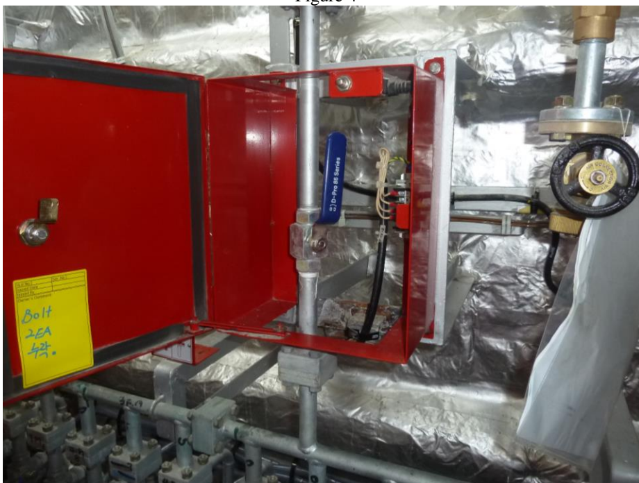
Ball Valve Box for cargo hold open shows operating lever and micro-switch for alarm
