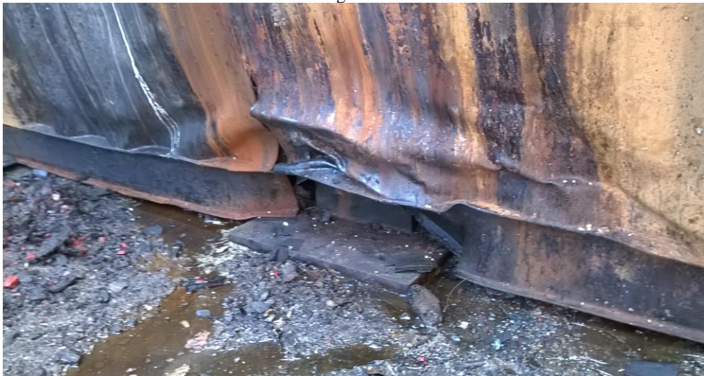
Base of container 70020 is torn on the cell locator as it is blasted outwards
