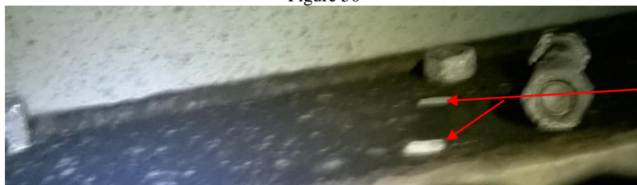
Nut and bolt moved to the right of original position revealing 2 areas of clean paintwork where it contacted the framing.
