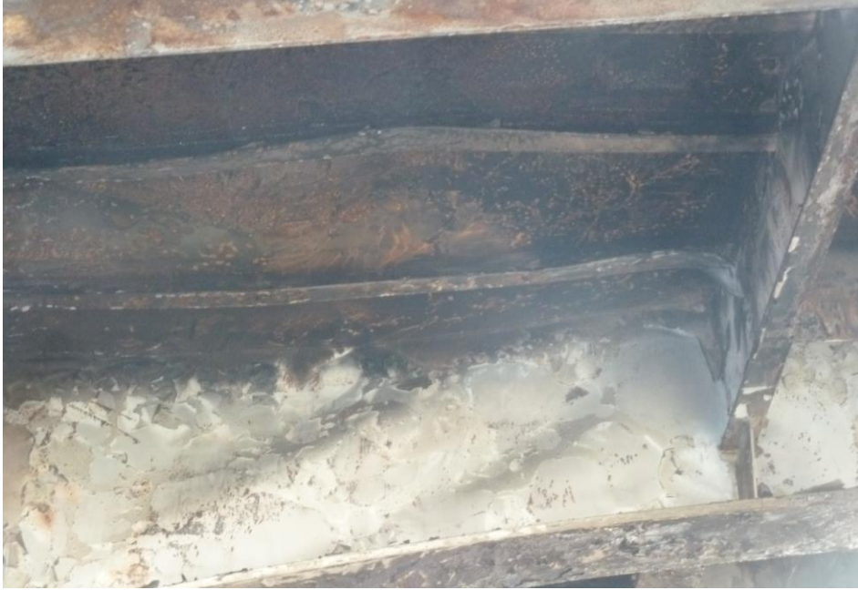
Heat damage to stbd inner hatch cover
