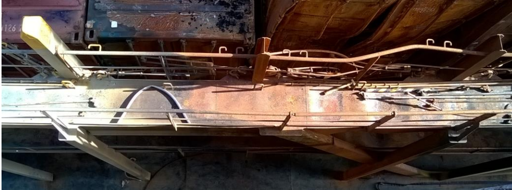
Damage to Lashing Bridge
