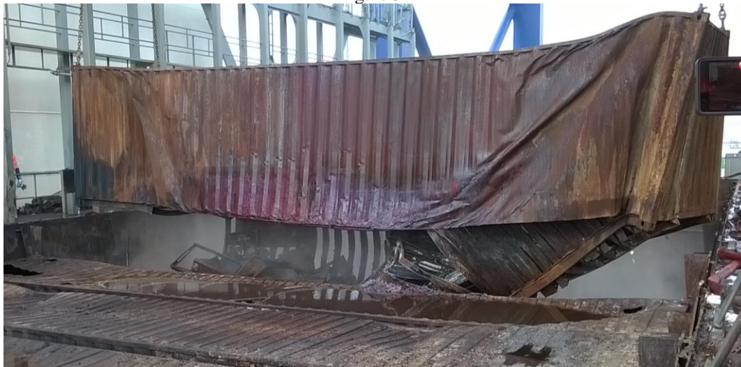
Container loaded directly above 700220 being lifted out loses the remnants of its contents which fall on top of 700220
