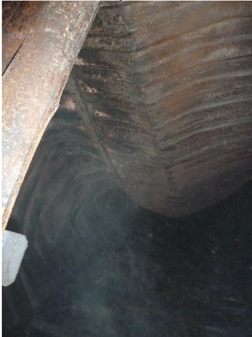
Container 700220 viewed whilst still in the hold, showing ceiling collapsed and sides blow out
