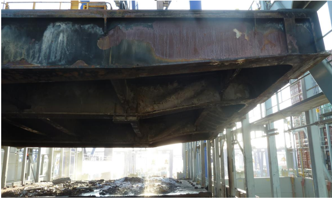
Bay 70 stbd inner hatch cover being removed in Algeciras
