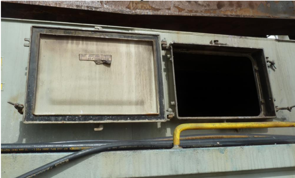
One of the manual natural ventilation flaps on the outboard side of an outer hatch cover
