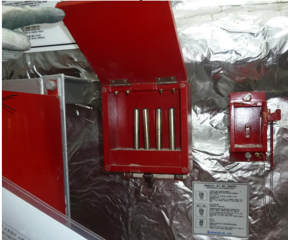
Manual lever box showing CO 2 bottle manual actuating levers
