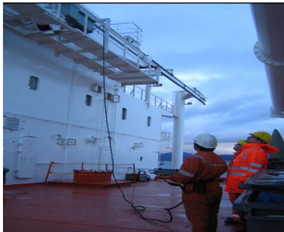
Gantry crane looking from port aft
