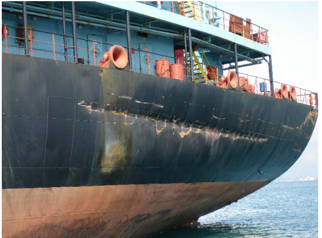
Side shell plating and associated internals at the aft port side shell were buckled 2m from the upper deck.
