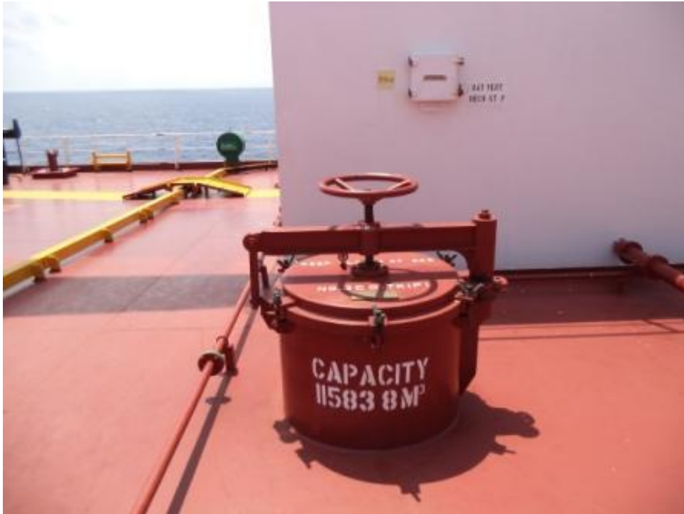
Sharp Lady – 3P Cargo Oil Tank – tank access hatch
