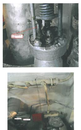
QCV blocked utilizing a bolt to hold in the open position. (Note: the painted portion on the bolt indicating possible long term condition.)
