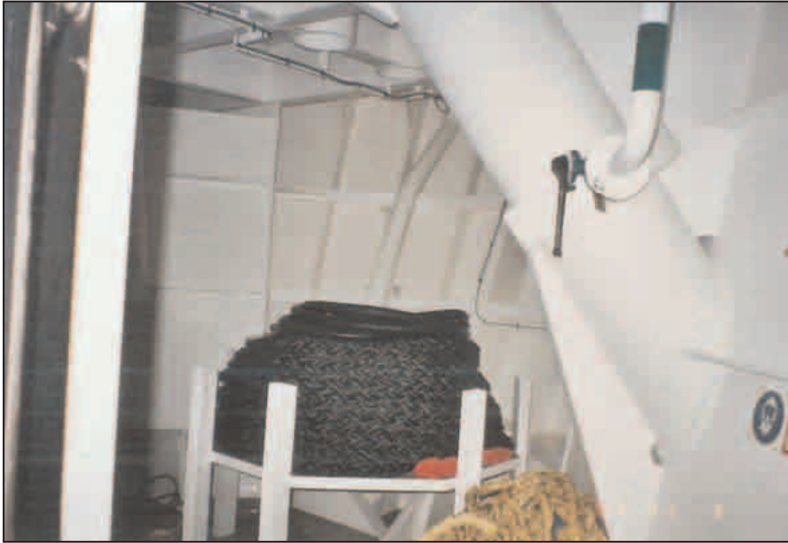
Forward store showing no internal damage
