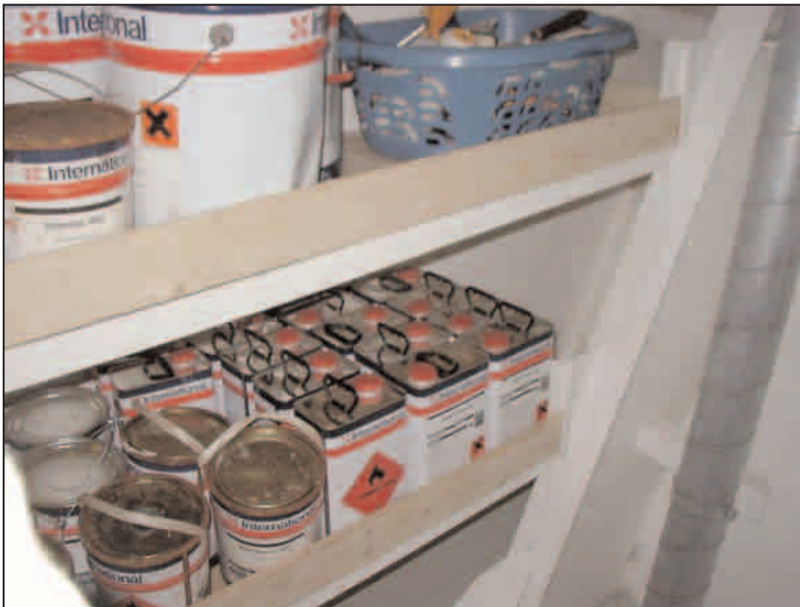
No damage internally to paint store
