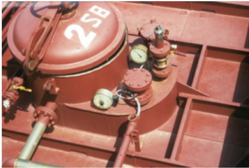
Fig 1. Example of Sampling and Ullage arrangements for each tank. (Behind is the open ullage port with the easy open handles in front is the restricted ullage / sampling port)
