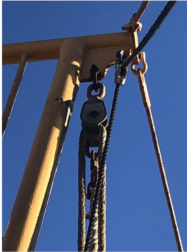
Fig 3 – Upper hauling block attached to port side of H frame
